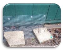
Trenching was not possible here, so the "L"- shaped mesh barrier is left aboveground. The mesh will be buried under rocks or soil
