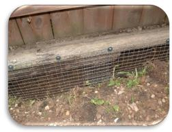
Welded wire mesh in a trench dug next to a fence that forms one side of a deck. The mesh is screwed to the deck using lath screws and fender washers. The trench is then back-filled with soil
