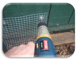
Attaching hardware cloth using a cordless drill/driver, lath screws and fender washers
